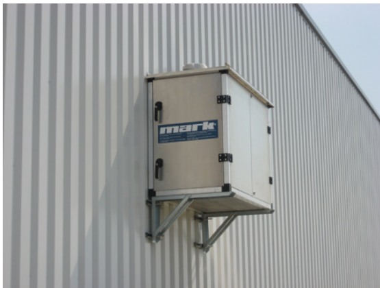
Option: burner outside the wall
